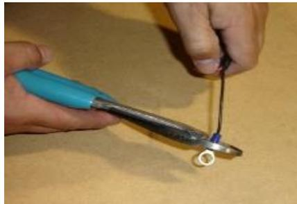
**13)** Crimp the supplied ring terminal to the BLACK wire and attach to the battery "-" terminal
